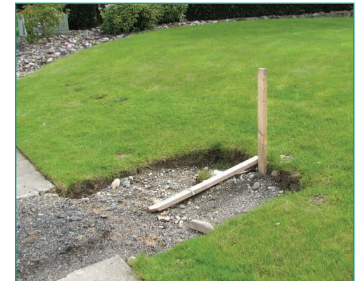
Example side sewer stub: Property owners will need to build a side sewer from their building to the stub in the street.
